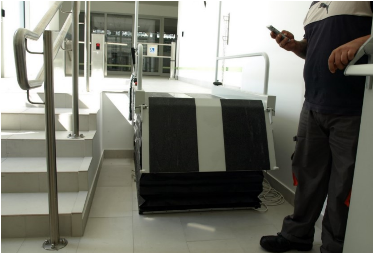
Fig. 2- Testing of an assistive device in an audit's on-site survey from the aspect of accessibility, Túskecsarnok, 2016. Source: ETIKK
