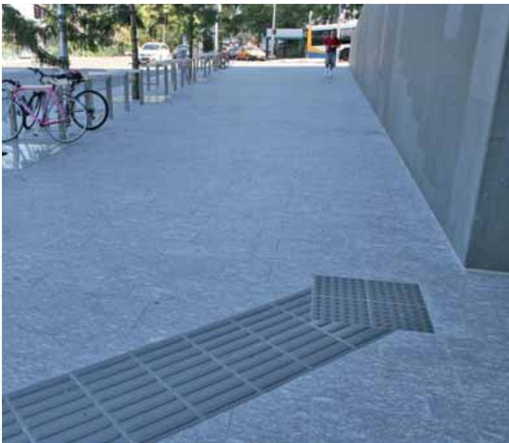
Figure 6 Tactile wayfinding trail and shoreline
