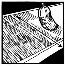
Make sure the broom strokes are perpendicular to the slope of the ramp.
